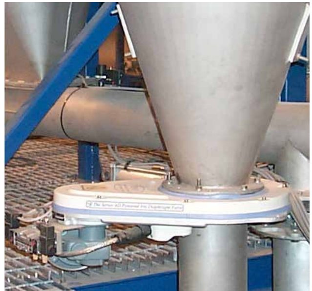
Mucon A2P provides inline control of product feed.
